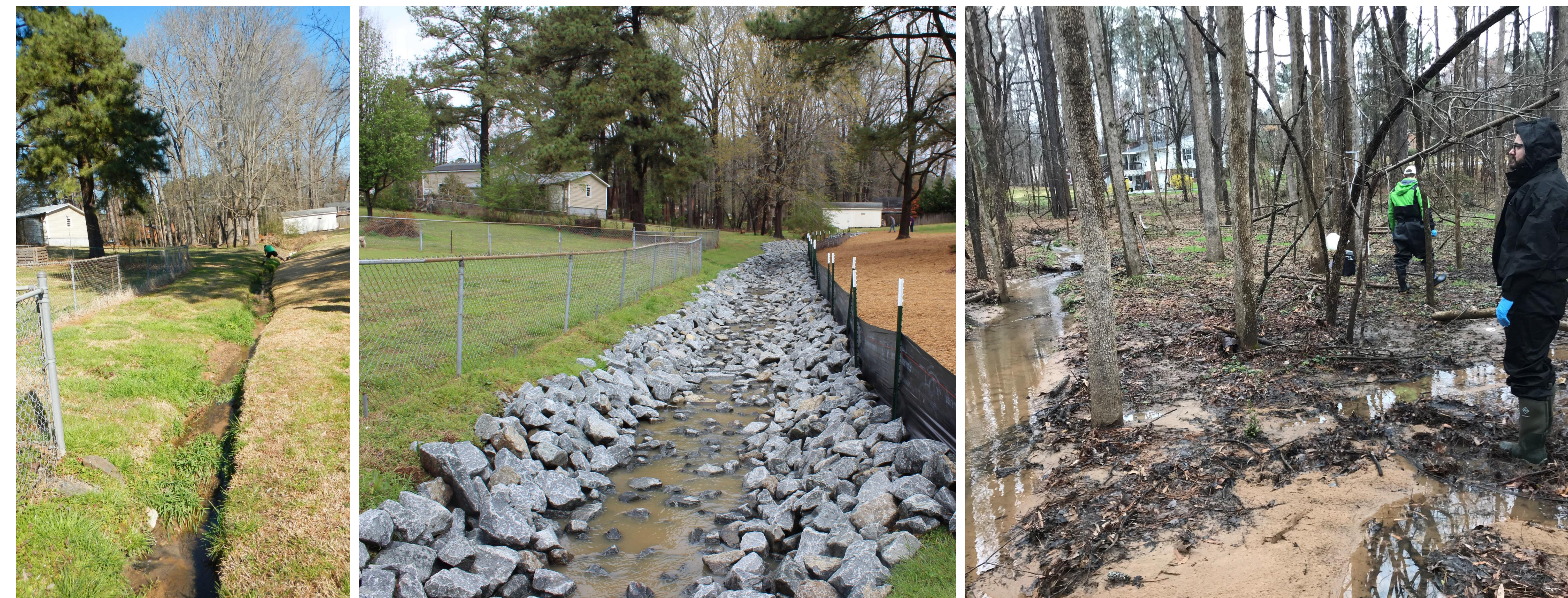
Figure 4. Photos of the stream before (left) and after (middle) the in-stream bioreactor was constructed. The photo on the right shows the natural wetland during a winter season.
