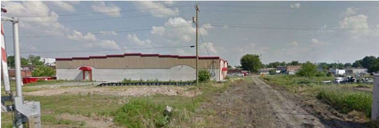
North Side View
