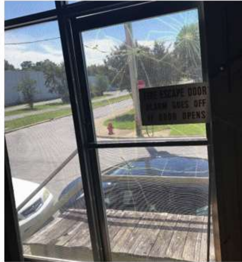
VIEW OF W 11 TH STREET OUT OF BACK ENTRANCE
