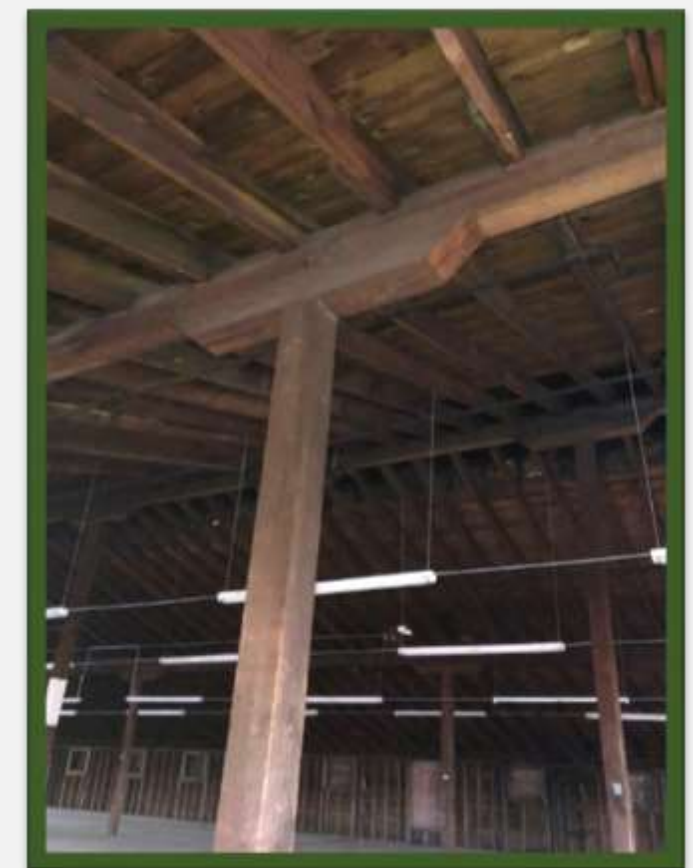
Photo 3: Structural elements that cannot be removed.
