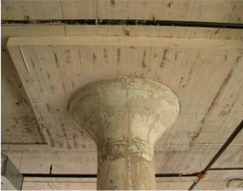
Currently, the space for the client is stripped to the building structure. Only vital building systems are in place. Large columns, on 22 foot centers, are located throughout. These columns are 2 feet in diameter and have a capital that cones out to a diameter of 5 feet. The capital supports an 8 foot square concrete platform used to help distribute the weight of the floor above.
