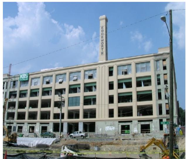
The Edgeworth Building renovation was begun in the late 1990's in three phases. The first phase involved the upgrading of the building structure and infrastructure. Phase two included the fitting out of the interior spaces for the prospective tenants and the construction of a parking structure rounded out phase three.
