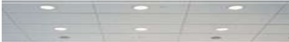
Acoustical Ceiling Tiles
