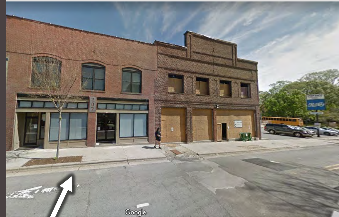
Right of building
