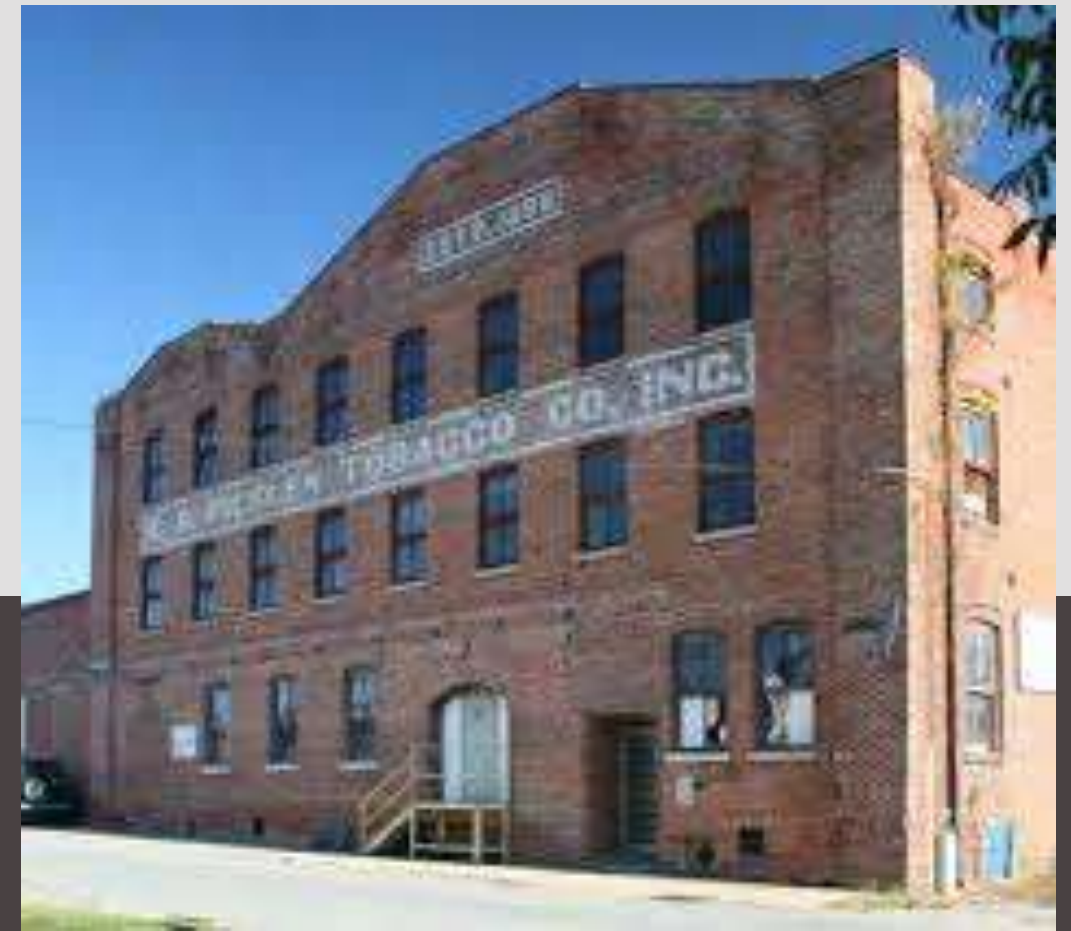
Historic Tobacco Warehouse in Greenville
