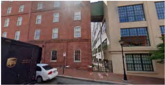
NORTH SIDE VIEW
