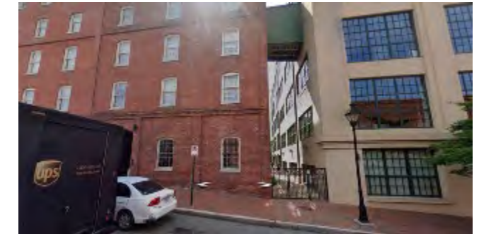
NORTH SIDE VIEW
