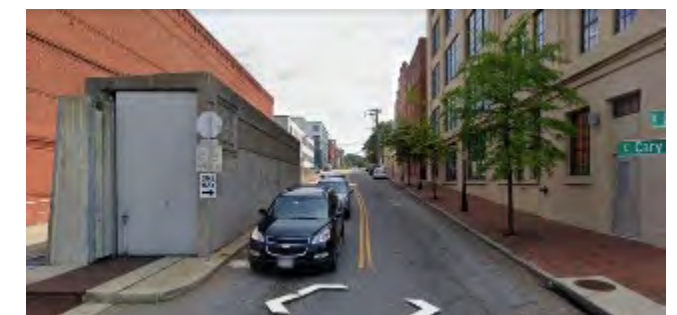
WEST SIDE VIEW
