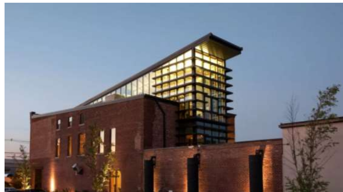
The Green Building in Louisville was a former dry goods store
