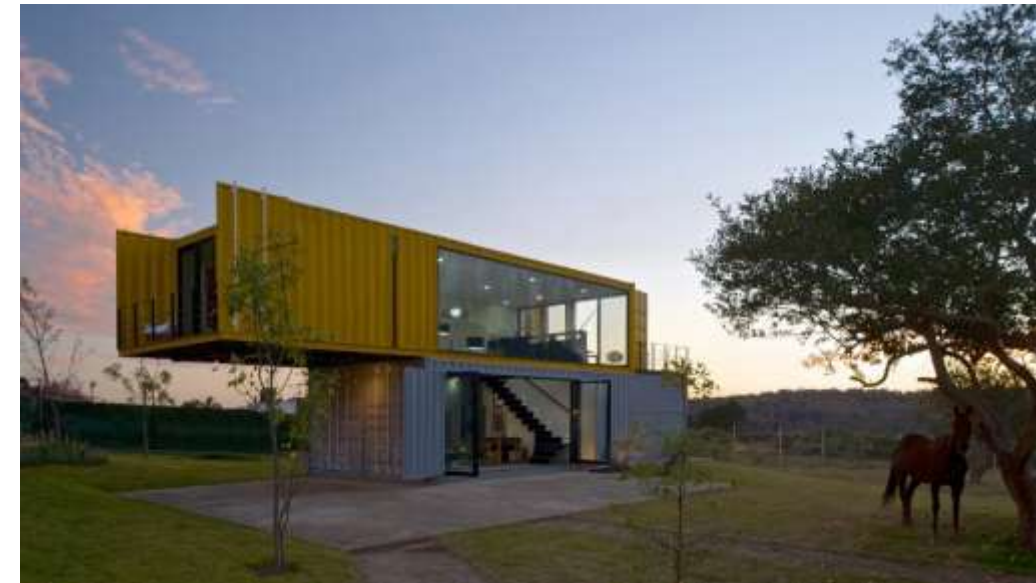
Two-story home constructed by stacking recycled shipping containers
