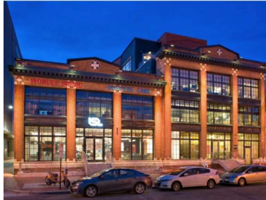
The former Wonder Bread Factory in Washington D.C. kept the original signs after it was redeveloped into offices
