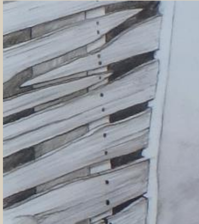
Plaster and Lath
